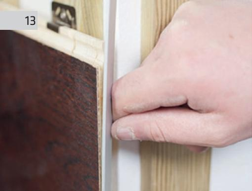
Then glue in an aluminium flat bar, for example, at this point, which serves as both decoration and protection on the sharp trimmed edge. Aluminium or wooden angle bars can be used instead.
