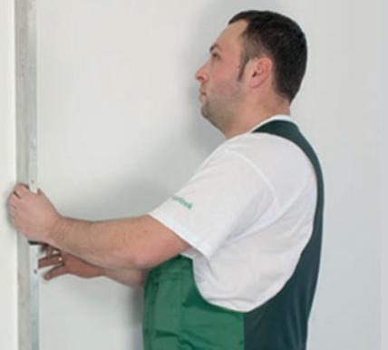
Check the level of the wall using a spirit level. The deviation must not exceed 2 mm over 2 metres.
