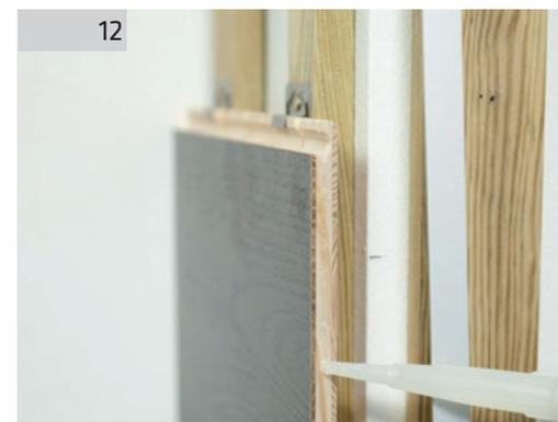
Apply assembly glue where the boards meet at the corner trimmed in this way.
