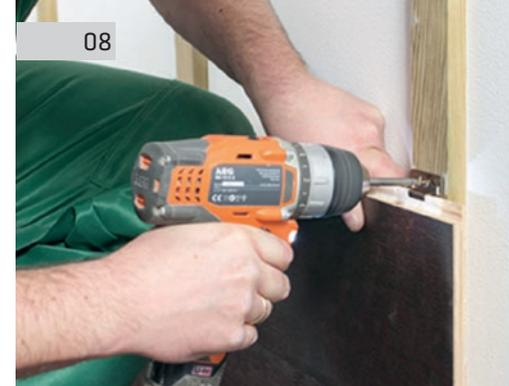
Apply wood or construction glue to the wooden structural beams (to a height of one board). Lay the first board, with the tongue removed, to the glued grid and fix it from above with the clips.
