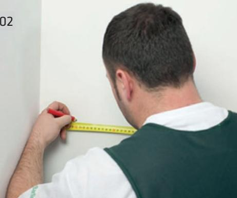
Mark the places where the wooden construction floats, with a cross-section measuring at least 18mm x 50mm, are to be attached. Attach the first float a maximum of 10cm from the internal or external corner.
