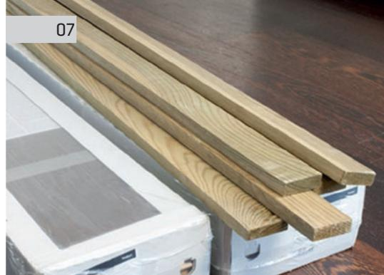
Before fitting the boards, acclimatise them in their factory packaging for around 48 hours. The Barlinek board is made from natural wood, which makes its pattern unique. Because of this, select and decide on the colour scheme of the surface to be covered before starting.
