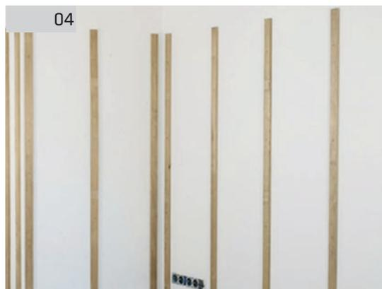
Attach the floats using rawlplugs, remembering that their heads must not protrude beyond the float.
