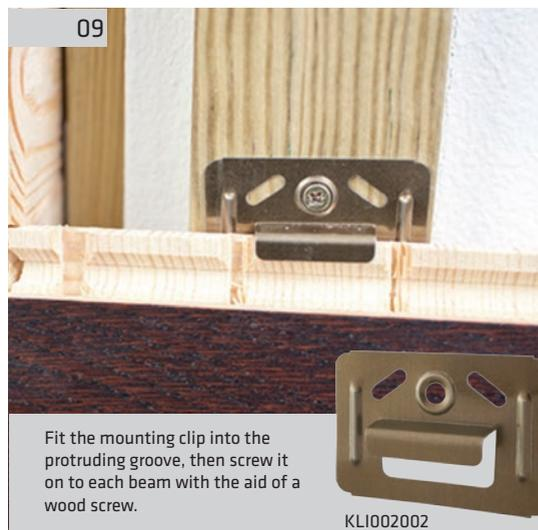
Fit the mounting clip into the protruding groove, then screw it on to each beam with the aid of a wood screw.
