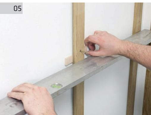
The floats must form a single plane. Check this by using a spirit level applied over a width of at least 3 floats. If necessary use plywood or other material to level the structure.
