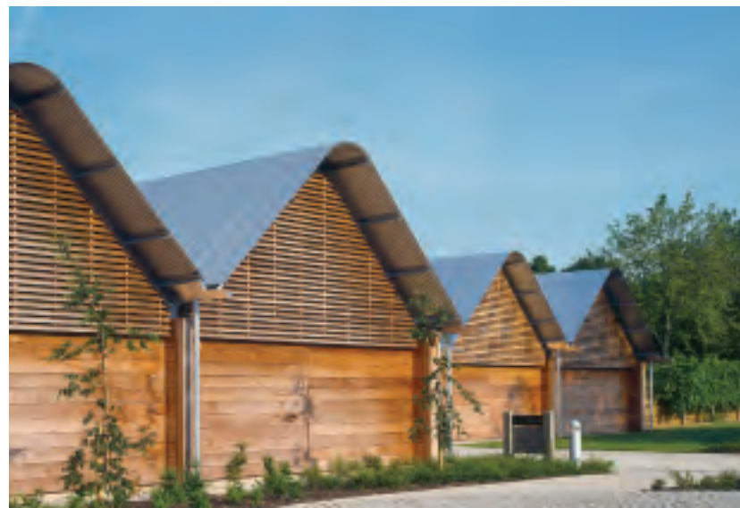
Partial elevation of cedar louvers
